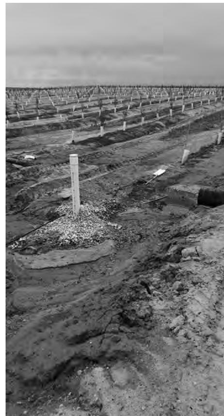
*So THAT'S a dry well ... The concept is very simple: instead of letting storm water run off to the ocean, the dry well directs the water down to the aquifer where it can recharge vital groundwater supplies.*
