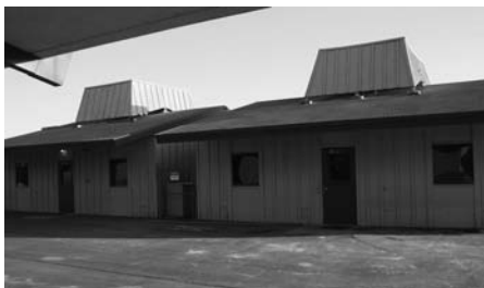
Old temporary classrooms were removed ...
