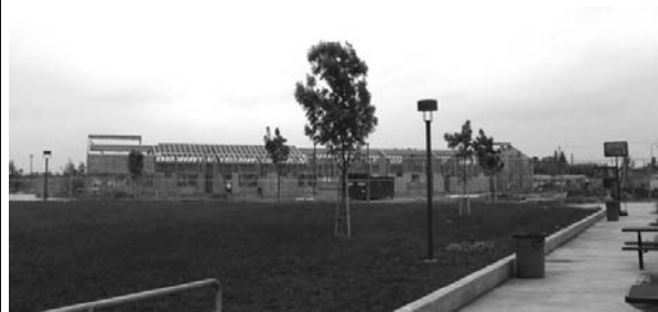
Liberty High School Phase II Classroom Wing.
