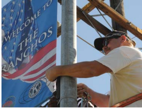
Travis Hart attaches one of the new welcome banners to a pole along Avenue 12. The banners were a joint project of the Ranchos Kiwanis and Golden Valley Chamber of Commerce.
