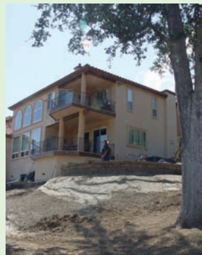
The steep slope on Harry Andris' home made conventional concrete impractical.
