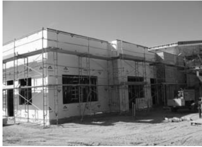
The work at Ranchos Middle School is progressing right on schedule.
